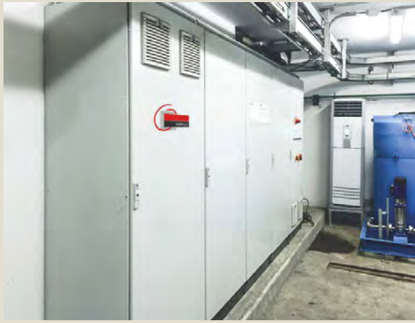
Figure 2: Full automatic prevention explosion protection system including monitoring and control, CO 2 storage tank and distribution
