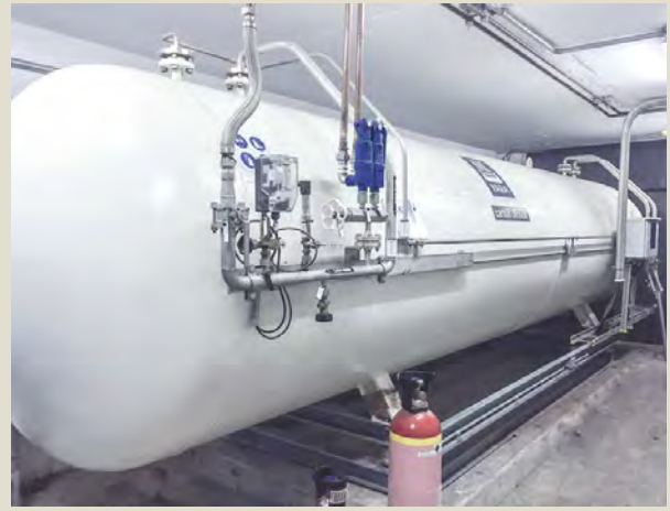
Figure 2: Full automatic prevention explosion protection system including monitoring and control, CO 2 storage tank and distribution
